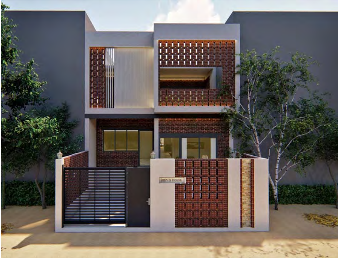
NARINDER JOSHI'S RESIDENCE, PILANI, RAJASTHAN
